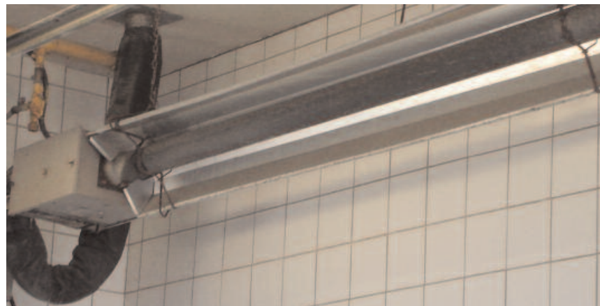
Figure 5.2 - Radiant tube heater
