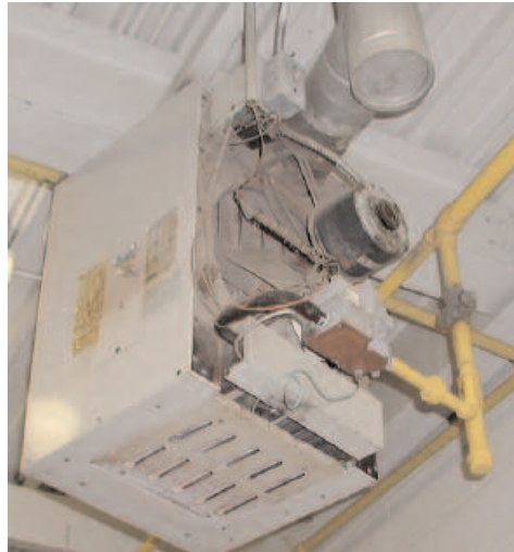
Figure 5.3 - Typical suspended unit heater
