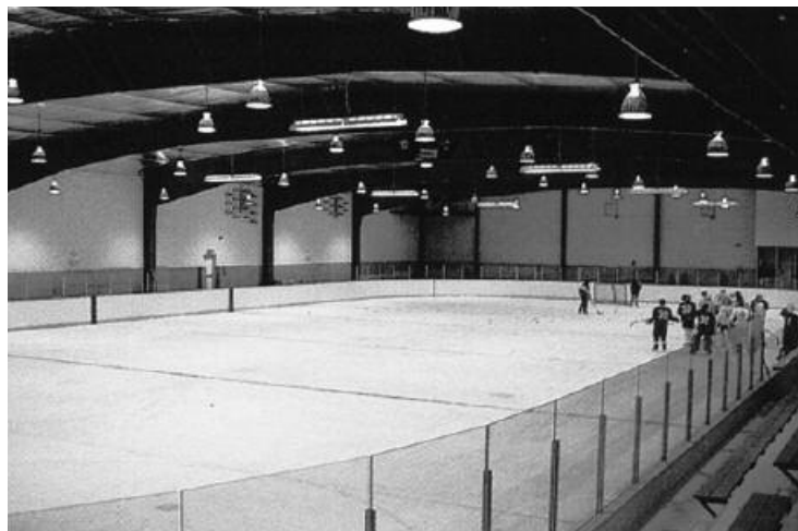
Figure 8.2 - Heat from arena luminaires
