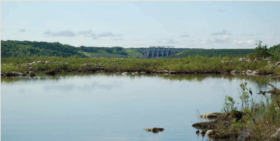
E.B. CAMPBELL HYDROELECTRIC STATION
