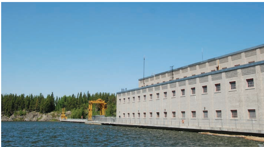
THE ISLAND FALLS HYDROELECTRIC STATION CONCRETE REHABILITATION PROJECT WILL EXTEND THE LIFE OF THIS 90-YEAR OLD SOURCE OF RENEWABLE GENERATION BY 50 YEARS.
