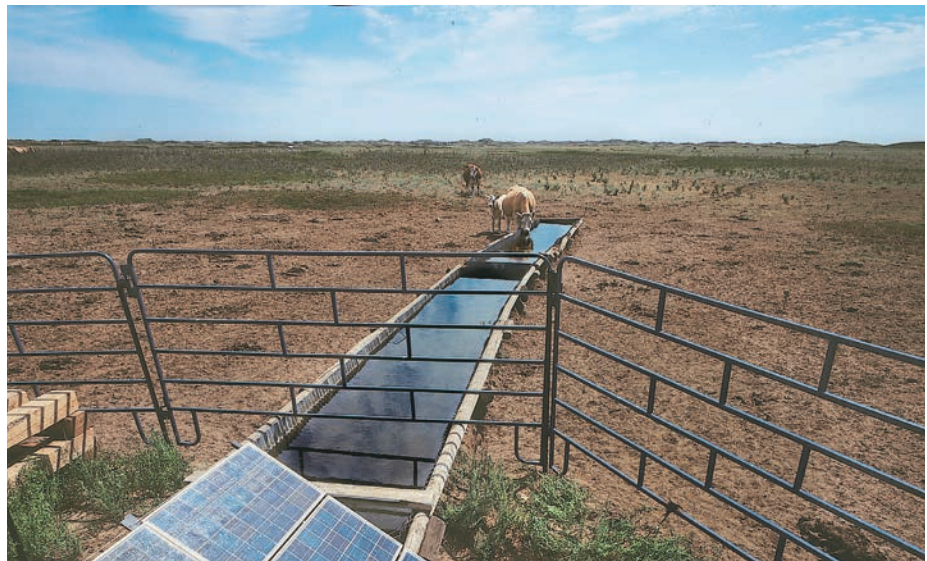
SOLAR INSTALLATIONS ARE GROWING IN SASKATCHEWAN IN STEP WITH INCREASING CUSTOMER SELF GENERATION.
