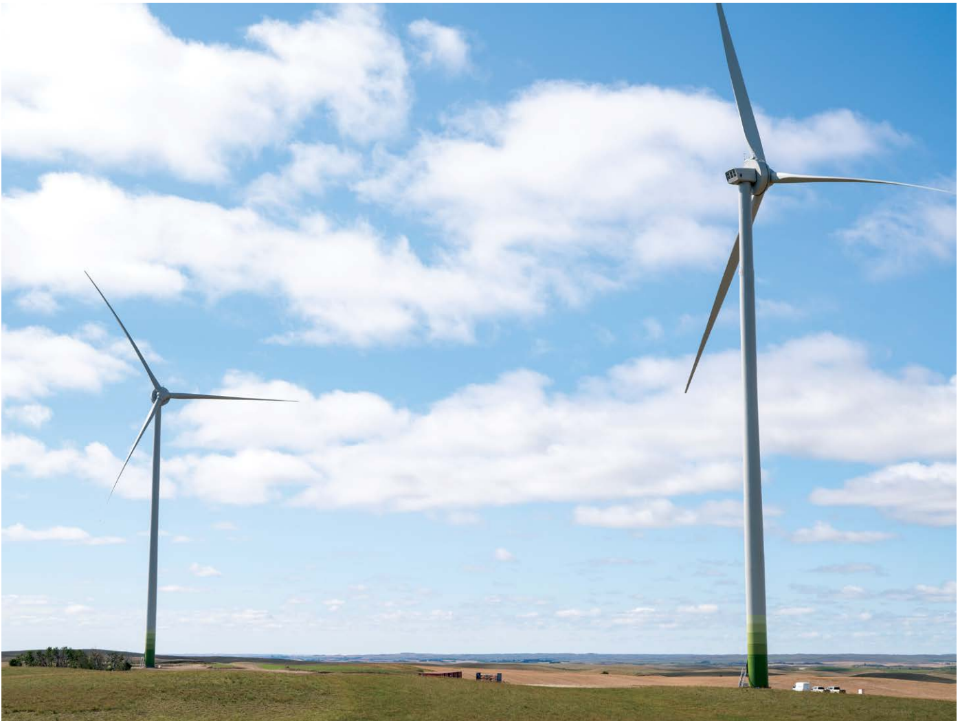
CAPSTONE INFRASTRUCTURE'S RIVERHURST WIND ENERGY FACILITY, LOCATED SOUTHWEST OF RIVERHURST, WILL SUPPLY SASKATCHEWAN WITH 10-MW OF WIND GENERATION CAPACITY WHEN COMPLETE IN 2021-22.
