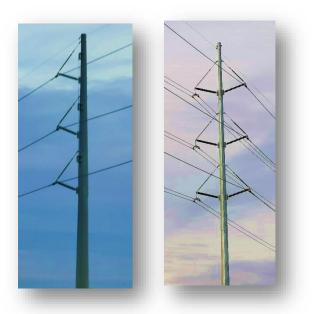
The picture on the left shows an example of a single-circuit structure with all phases of conductor on one side of the structure.
