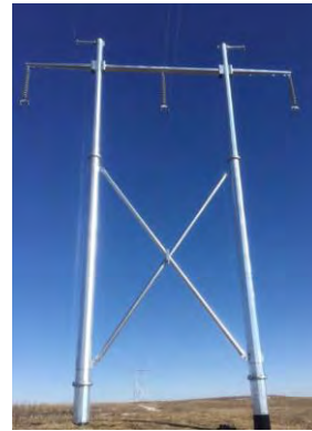
230 kV Single-Circuit Galvanized Steel H-Frame Structure
