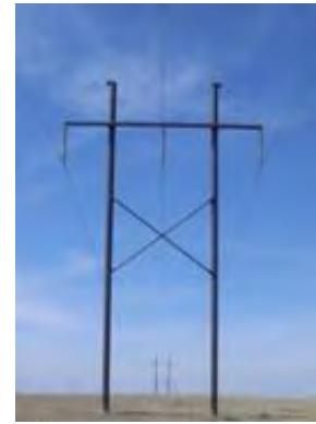
230 kV Single-Circuit Tubular Steel H-Frame Structure
