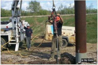
Installing ground rods
