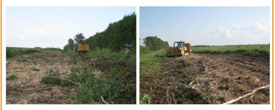
Drum mulcher clearing right-of-way
