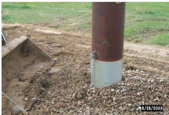
Crushed rock backfill
