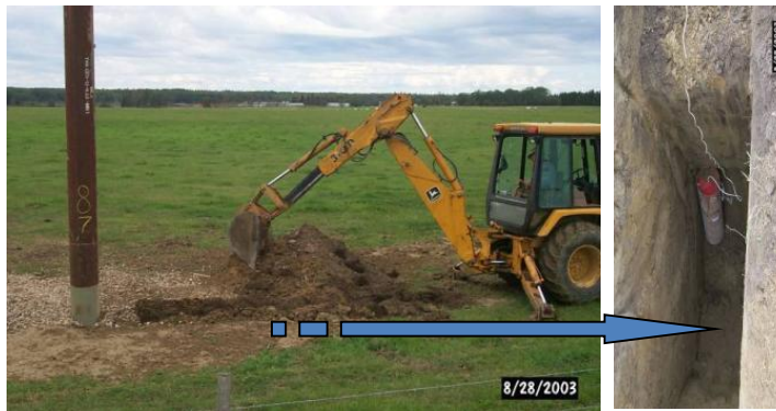
Installing sacrificial anodes
