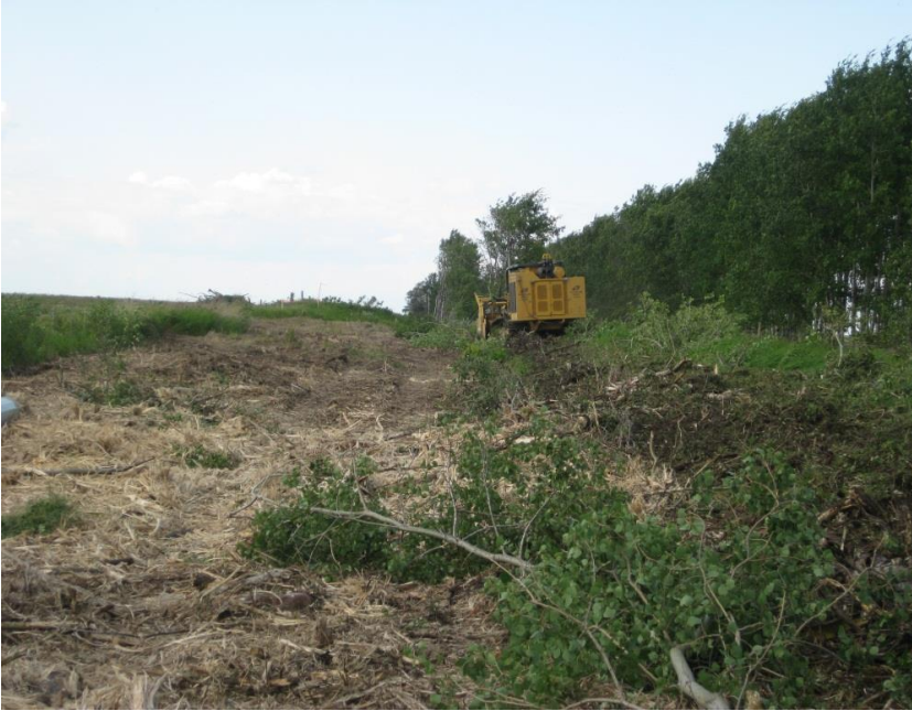
Drum mulcher clearing a right-of-way for a new transmission line
