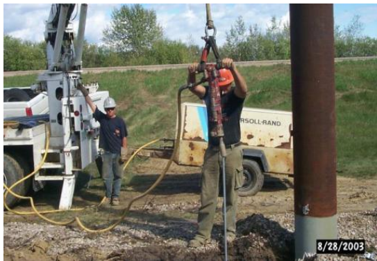
Installing ground rods
