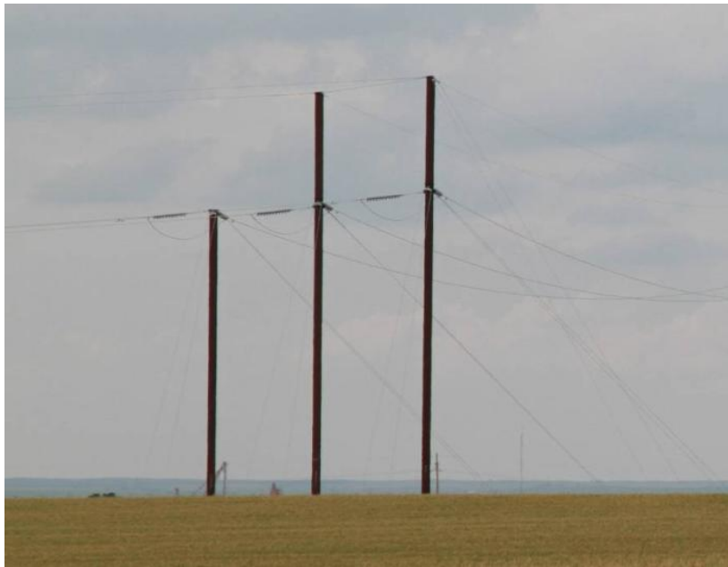
Heavy Angle Deflection Structure
