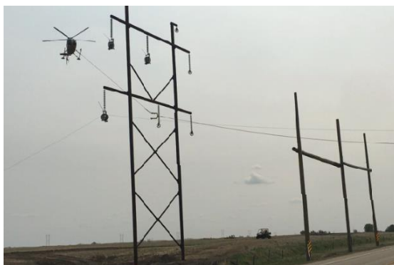
Helicopter Conductor Stringing
