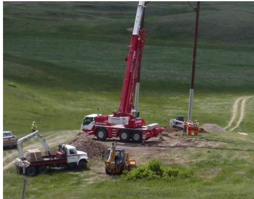
Temporary crane pad leveled for structure setting
