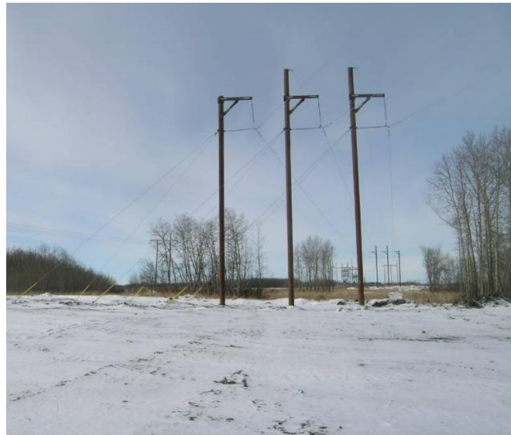
Medium Angle Deflection Structure
