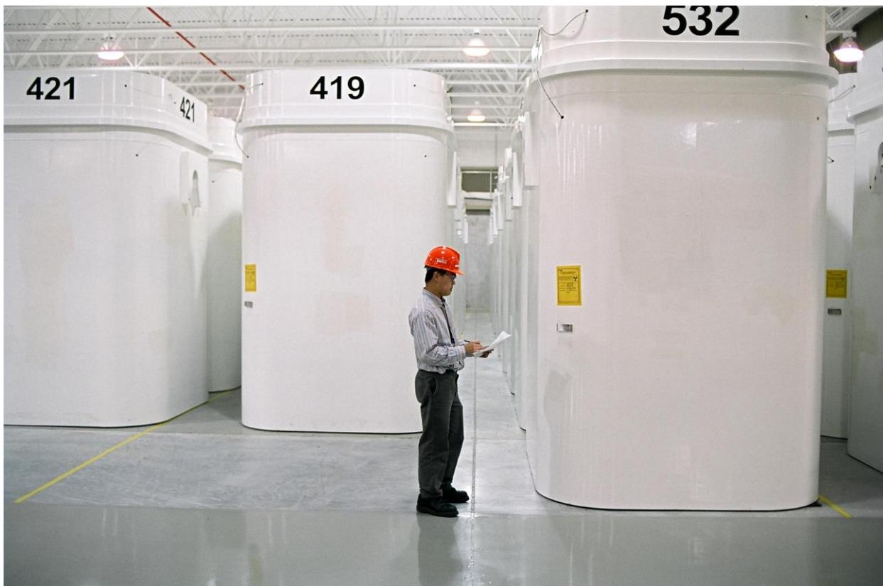
**Figure 3-3 Shielded dry cask storage example**
